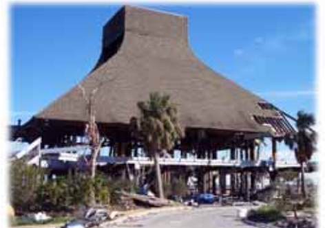
Diamondhead Marina and Yacht House after the storm.
